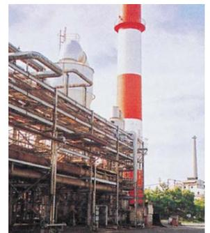
Desulfurization facilities attached to boilers at our Tokushima Plant
